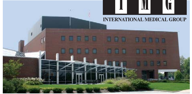
IMG World Headquarters, Indianapolis, Indiana
